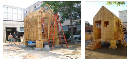
Figure 7 Full scale artifact under construction (a) and finished (b).
